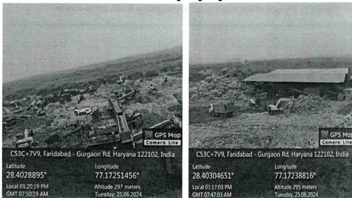
**Photo 3: Biomining with the use of a trommel**
